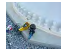
Tower flange connections
